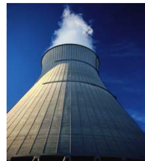
Figure 1: Steam rising from a stack.
