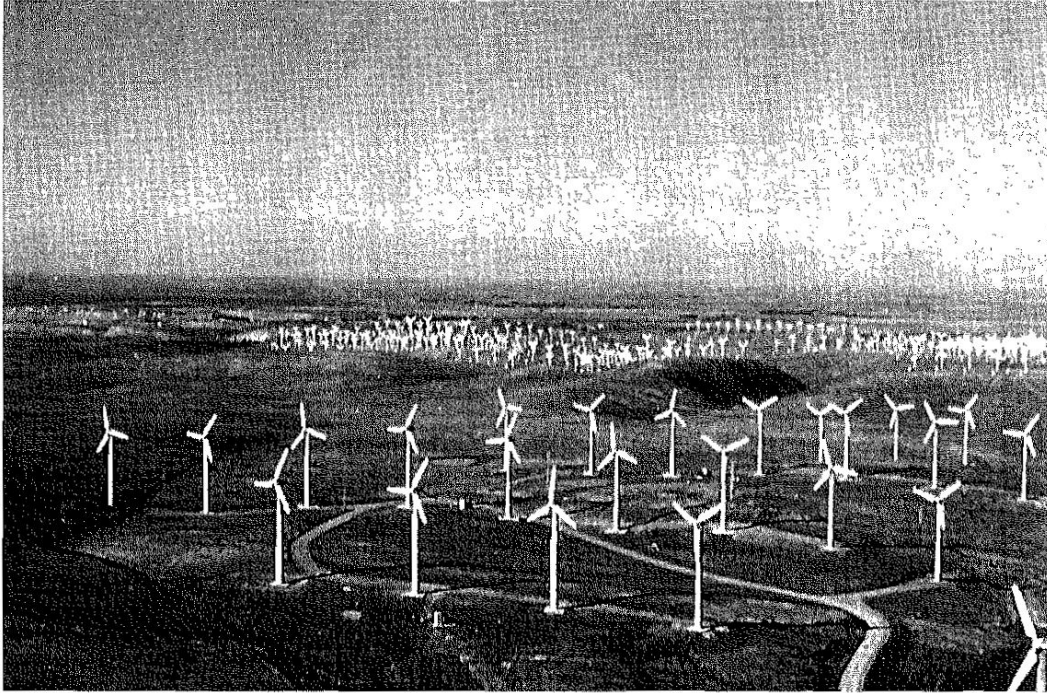
Figure 12.24: Wind farm located in Altamont Pass, near Livermore, CA. Maximum power output is 5 MW at a wind speed of 15 mph. Courtesy U.S. Department of Energy.
